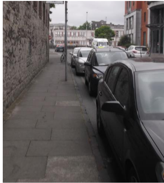
Figure 3.4 – Cracking and Reduced Footpath Widths on Streets Adjacent to Proposed Development
