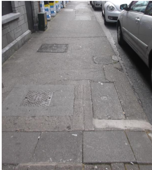
Figure 3.4 – Cracking and Reduced Footpath Widths on Streets Adjacent to Proposed Development
